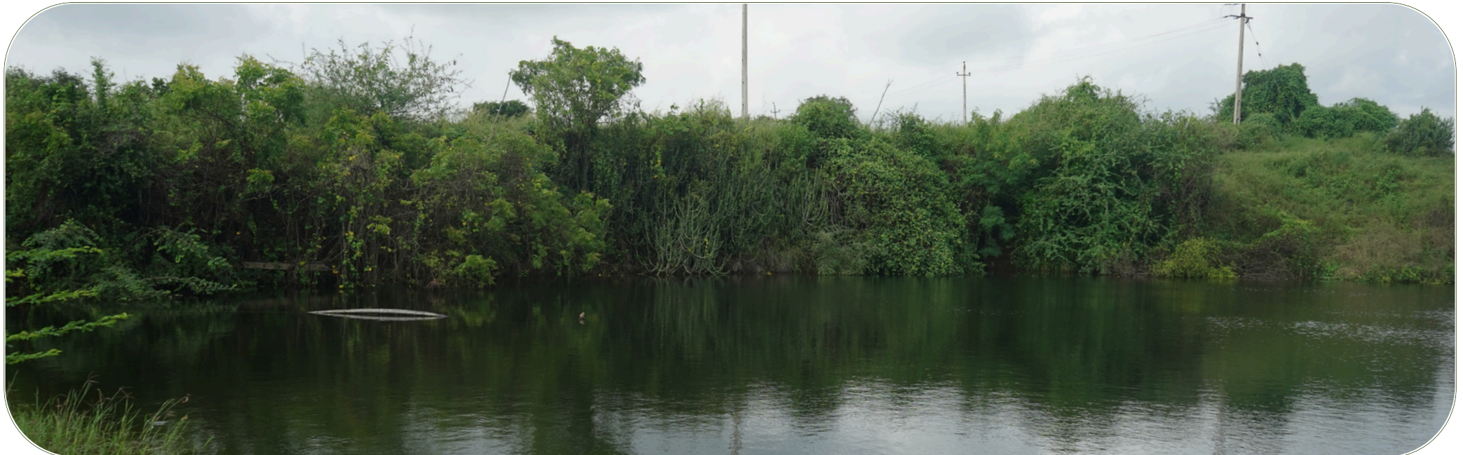
Restored reservoir enhancing water storage and improving water availability for local communities and agriculture
